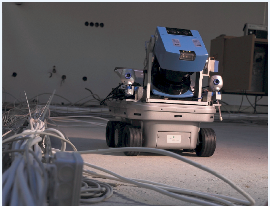
Figure 1: The autonomous mobile robot Kurt3D mapping a construction site.
